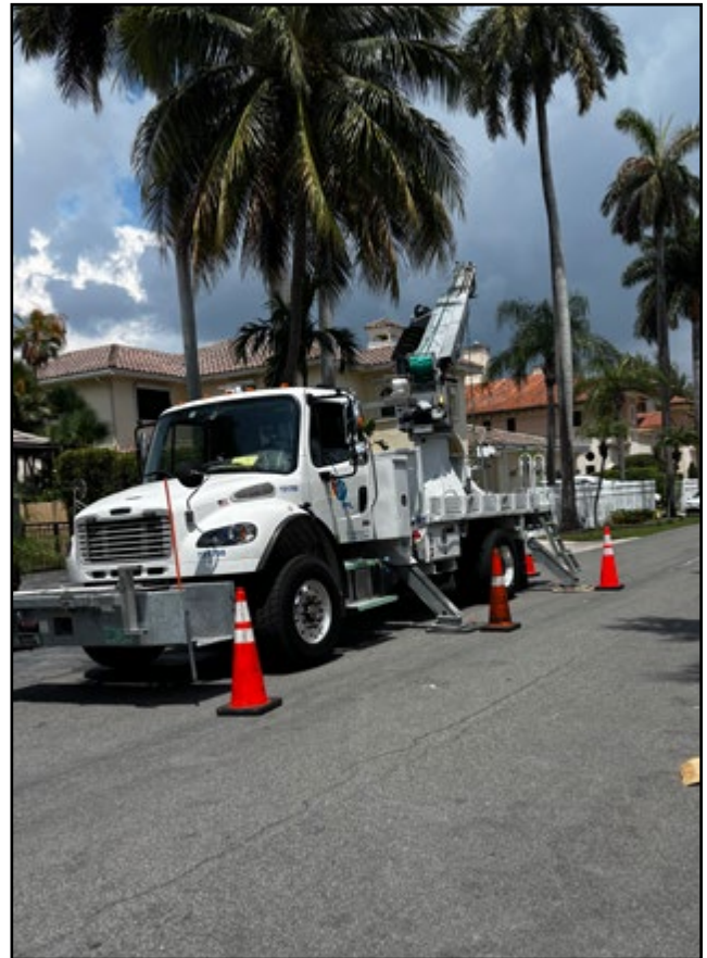
FPL Truck working on the problem
